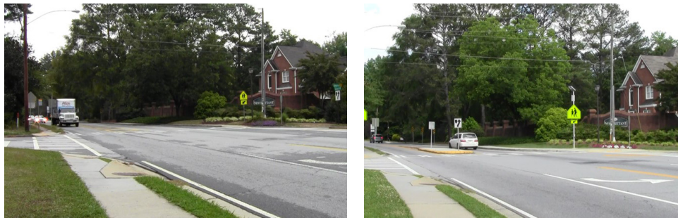
Figure 8. Ground-level view of the crosswalk at Torah Day School before (left) and after (right) the installation of the median, curb extension, and RRFB
